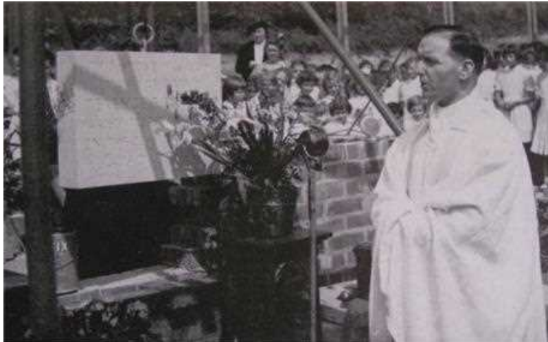
Father Tanner lays the foundation stone of St Ursula's new school: 1960 June 22nd (courtesy St Ursula's Community)
