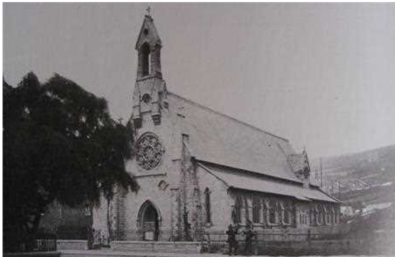
One of the first photographs taken of St Paul's Church, c1870 Note that there is no bell yet and the present presbytery and the apse East end had not yet been built
